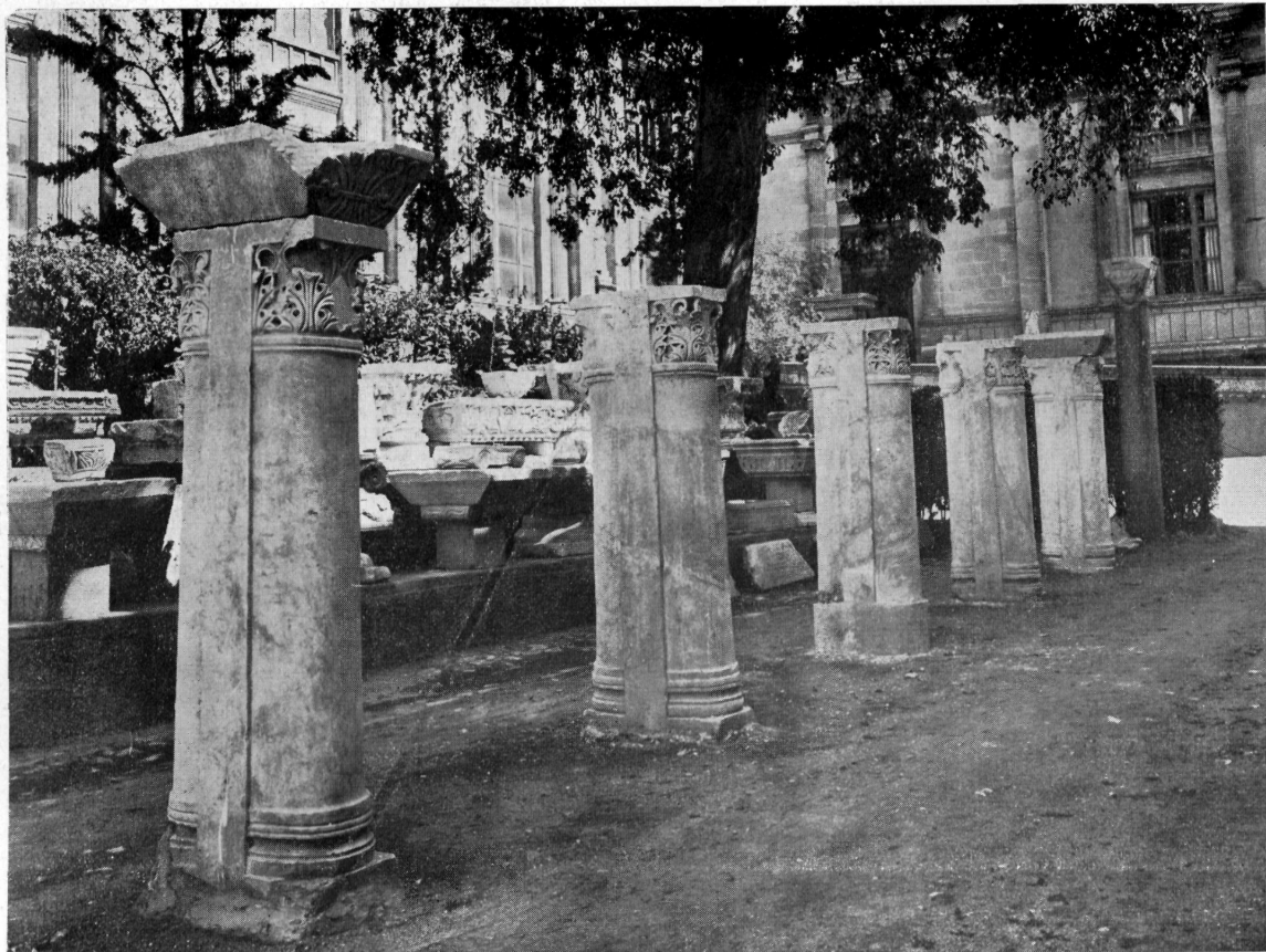
FIG. 6. — DOUBLE COLUMNS AND IMPOST CAPITALS FROM «BATH» BUILDING.
